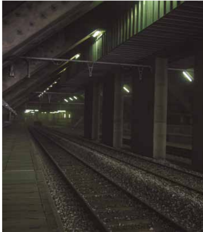
↑ TGV Tunnel (Brussels-Amsterdam Line Section) Antwerp, Belgium
