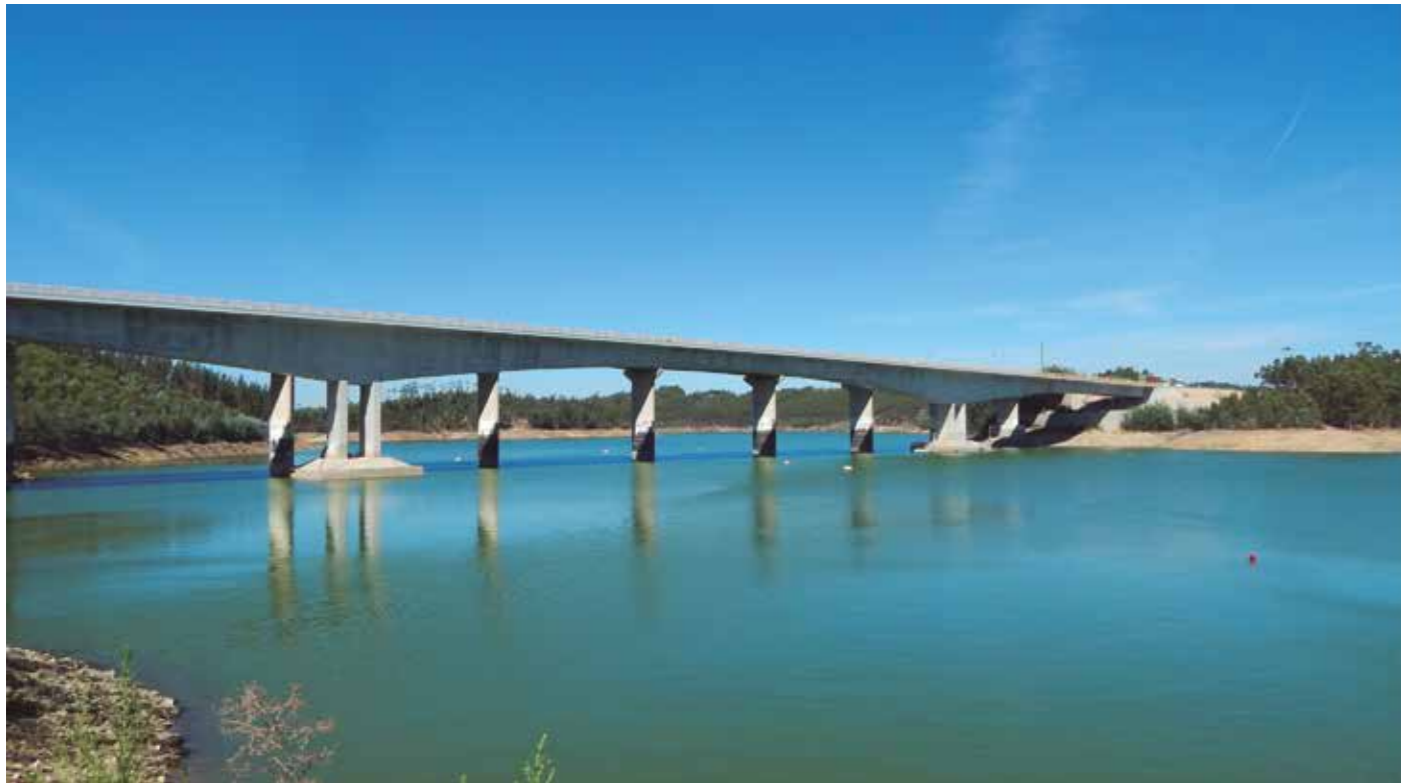
↑ IP3 — Bridge over Dão's river mouth Santa Comba Dão, Portugal
