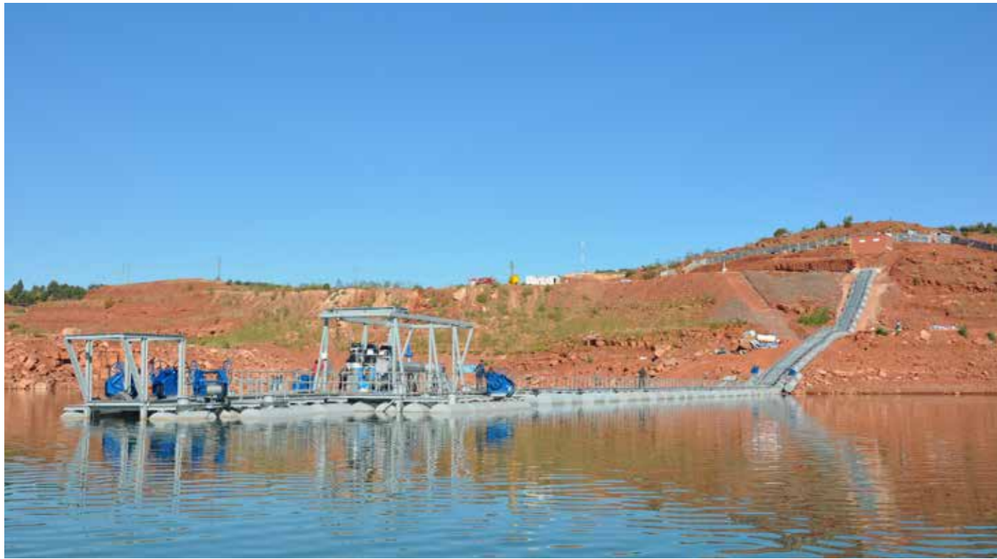
Water Catchment, Hâssan I Dam Azilal, Morocco
