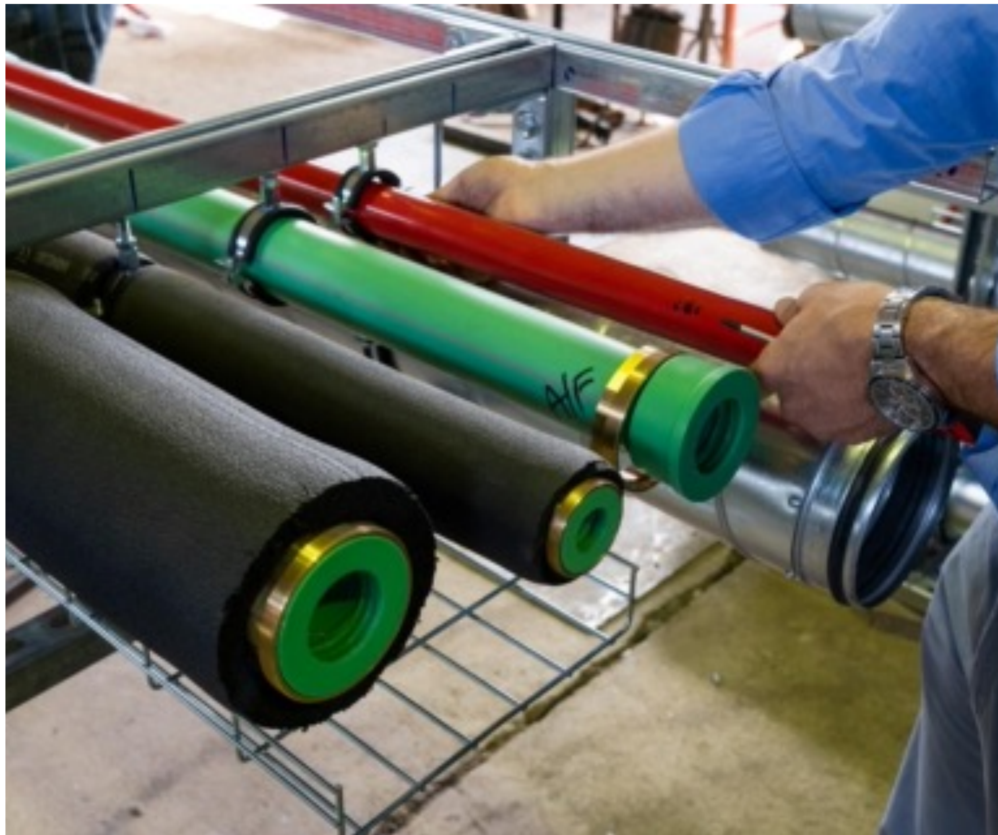
Fig.9 - Pipes, cable tray and ducts already assembled on the rack structure.
