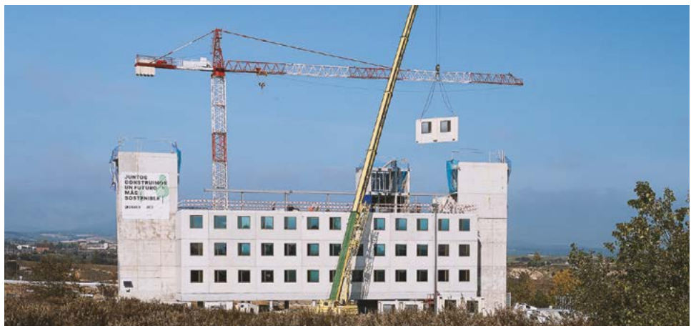
Assembly of Blufab industrialised façades
